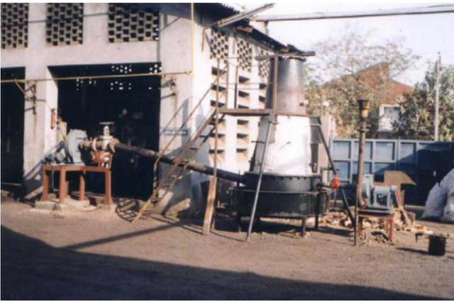
**Fig. 11.** Gasifier system for steam generation installed at Dinesh Pharmaceutical Pvt. Ltd., Nandesari.
